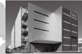
Industrial Mechatronics Systems Works/ Nagoya Works
