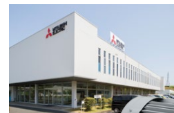
Nagoya Works, Shinshiro factory: 3-phase motor manufacturing factory
