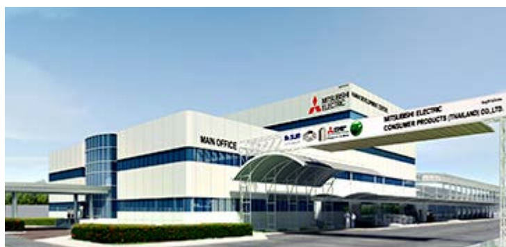
Mitsubishi Electric Consumer Products (Thailand) Co., Ltd.全景
