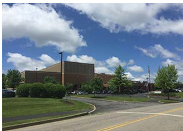
Mitsubishi Electric Power Products, Inc.
